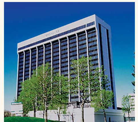
Metropoint Center for Business at I-394 and Hwy. 169 in Minneapolis.
